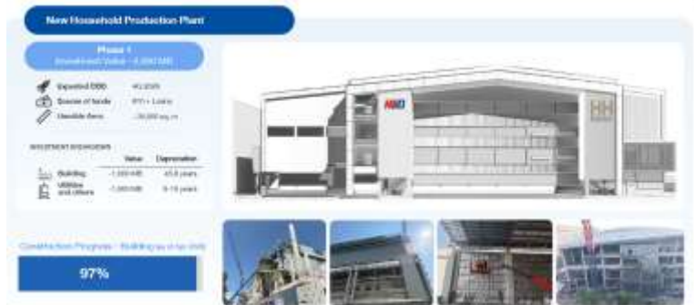
Fig 2: New Household Production Plant
